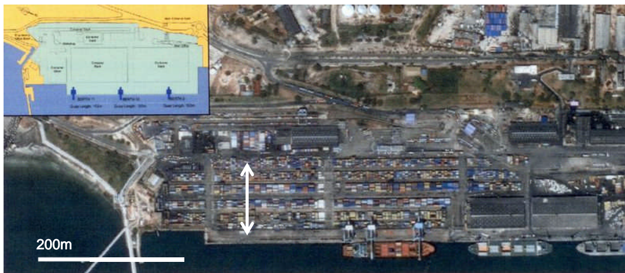
Figure 4-3 Narrow Back yard of DSM Port
