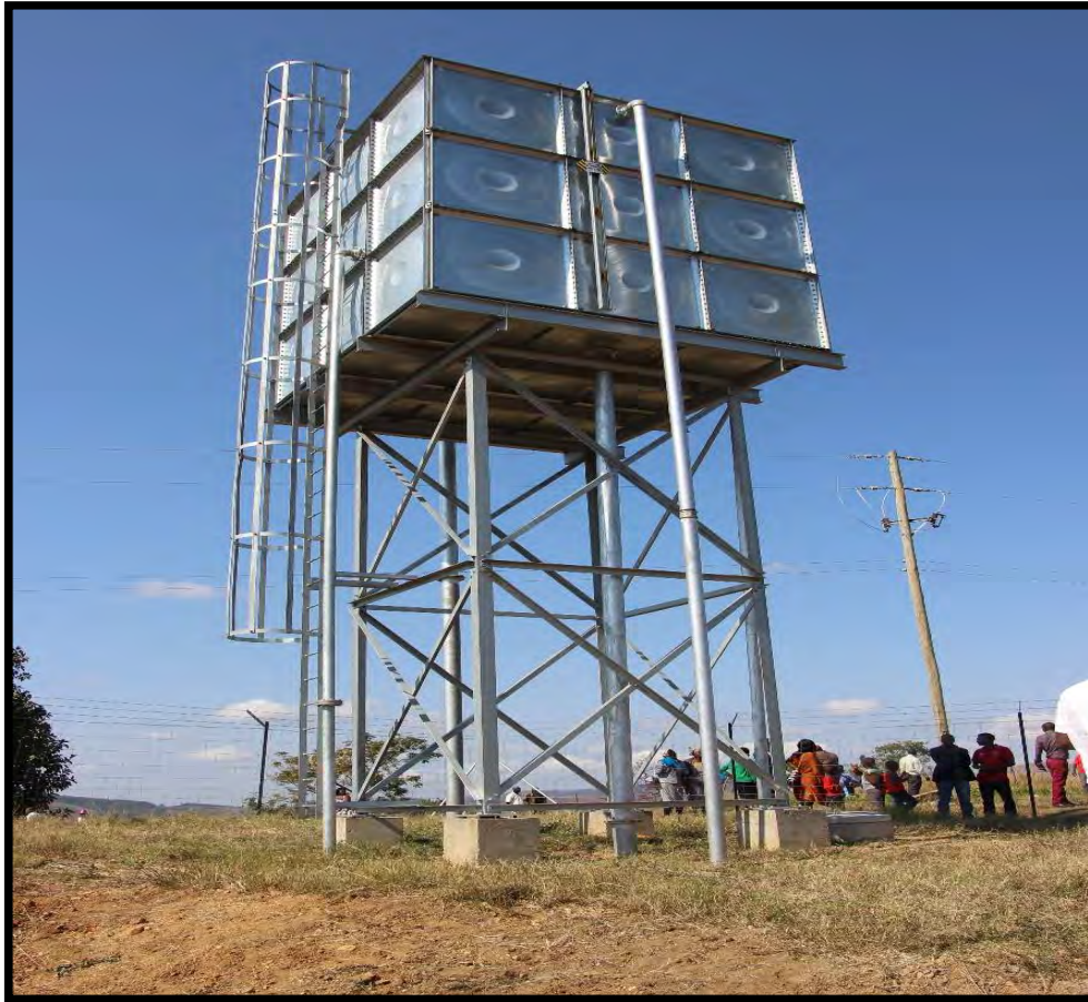
FIGURE 6 – AN ABECO TANK FOR POTABLE WATER SUPPLY
